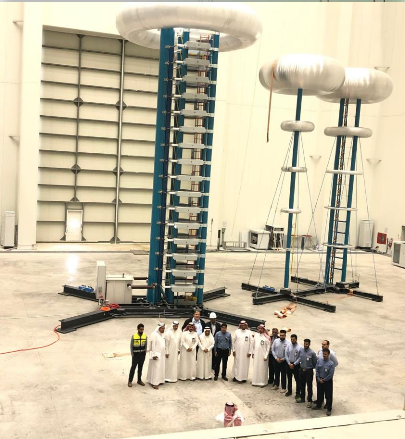
HV Testing Lab - (Project Completion Q4 2022)
