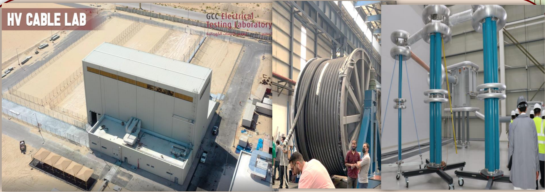
HV Cable Testing Lab - (Operational Q4 2021)
